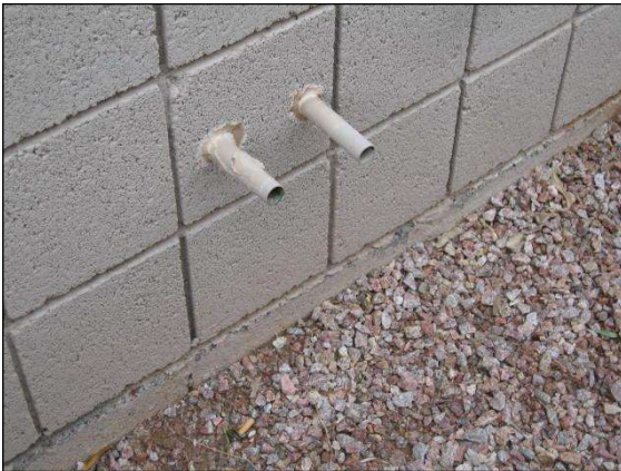
Figure 1: drains at site
