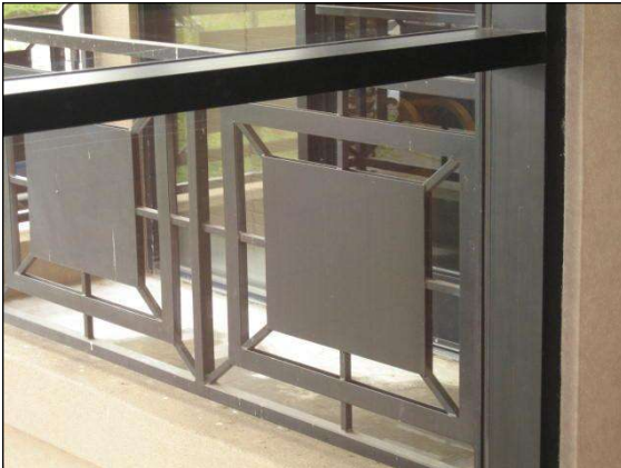
Figure 1: guard rails are servicable
