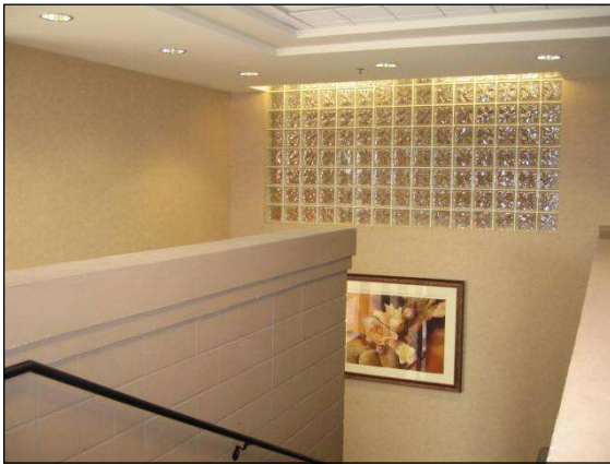
Figure 1: the stairwell, lights, rails and landings are in safe condition
