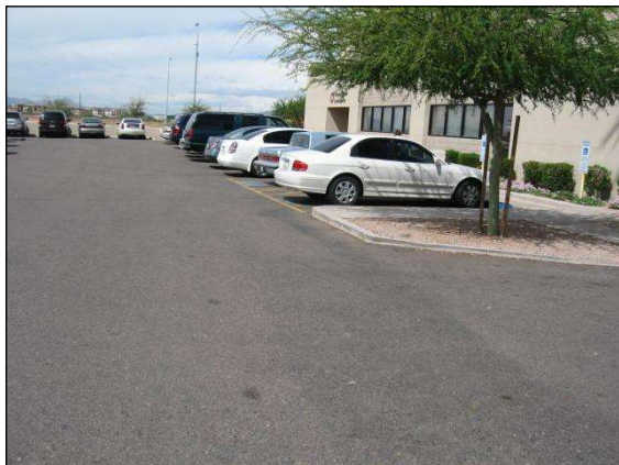
Figure 1: very few ADA parking spaces
