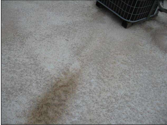
Figure 1: the roof has very little ponding due to good roof drainage.
