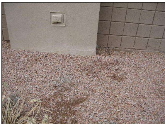
Figure 1: CMU wall with stucco build outs
