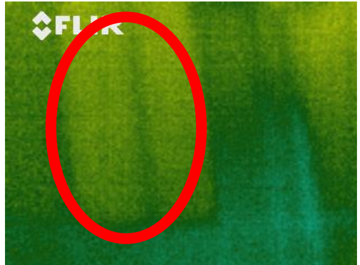
Location Floor: 2DN FLOOR Location Room: LOOKING AT SOUTH BEDROOM WALL
